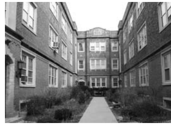
#14 TERRACE COURT APARTMENTS 6207 – Seventh Avenue (1928) Neo-Classical Revival
