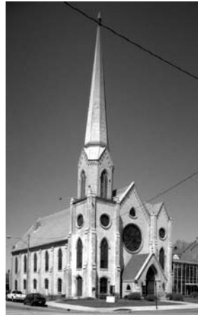
#24 FIRST CONGREGATIONAL CHURCH 5934 – Eighth Avenue (1874) Gothic Revival
