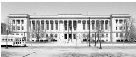
#2 KENOSHA COUNTY COURTHOUSE and JAIL 912 - 56th Street (1923-1925) Neo-Classical Revival
